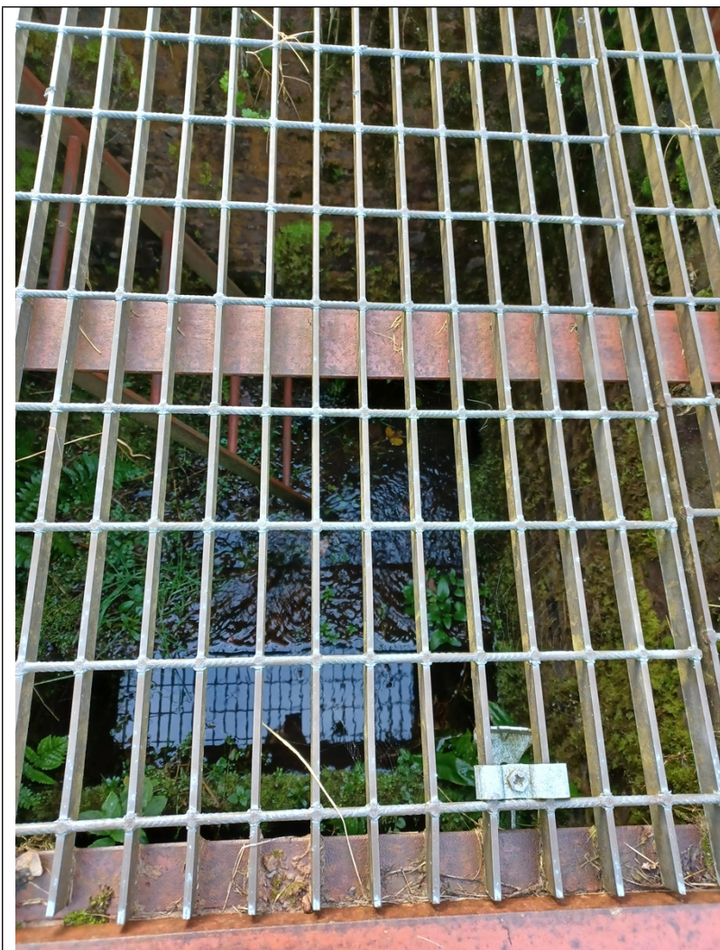
Image 3: Treated effluent for discharge
