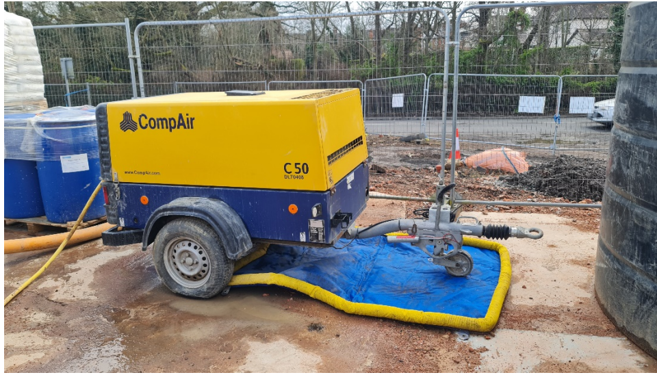
Figure 7 – Typical Mobile Plant including Engineered Containment System.
