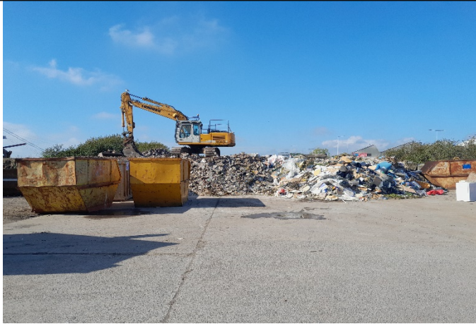
Photo 1 - Hard standing which was in good condition
