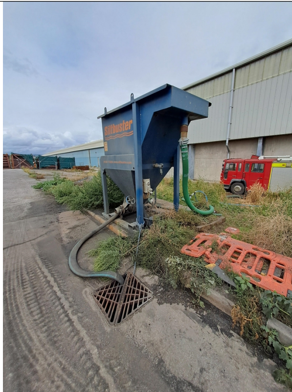
Figure 2 – The silt buster as observed during the visit.
