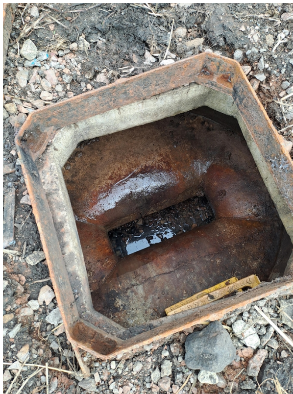
Figure 5 – The sample point chamber as observed during the visit.
