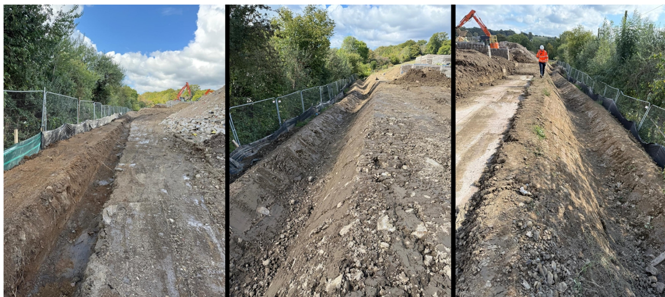
Figure 5 – Evidence provided by TW showing the works completed on the shallow surface grip.
