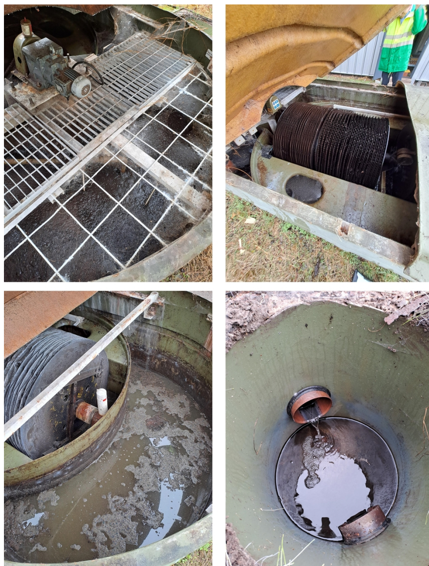
Figure 1 – The system chambers as observed during the visit.
