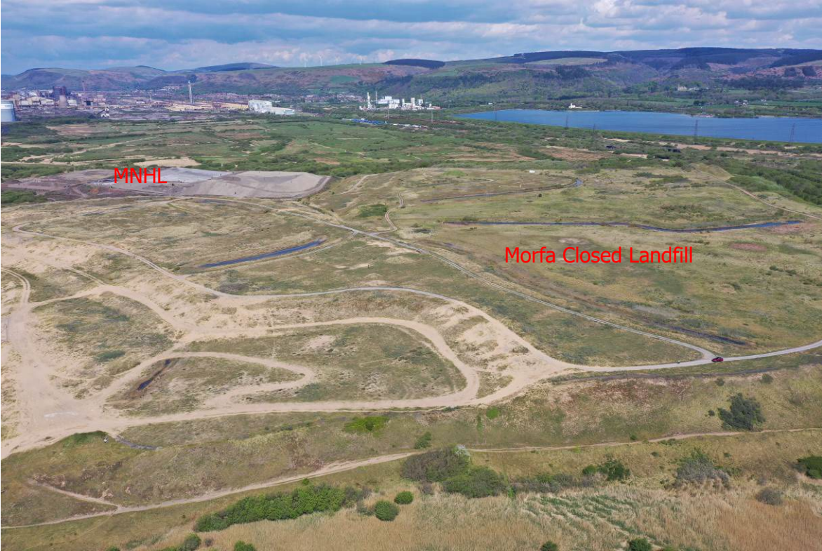
Plate 3-7 Typical restoration profile on surface of MCL
