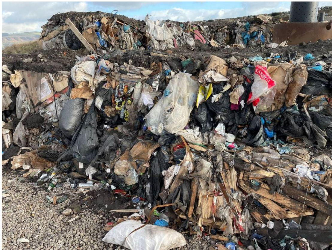
Plate 3-6 Typical waste placed in bio-cell beneath daily cover
