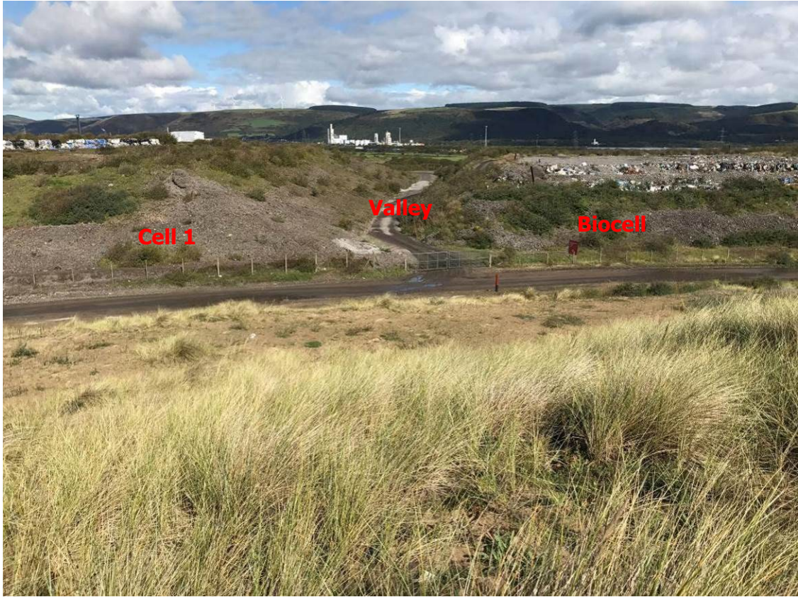
Plate 3-1 View north towards Non-Hazardous Cell 1 prior to re-profiling, valley feature and uncapped Biocell
