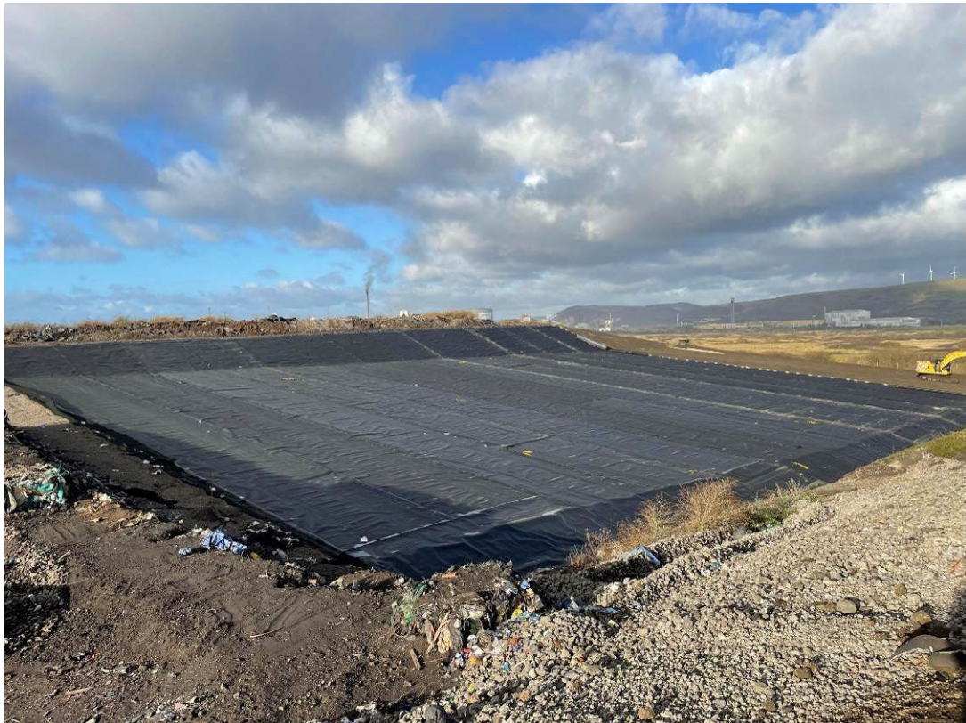
Plate 3-2 View north over new Biocell extension geomembrane lining
