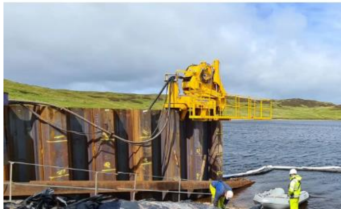
Fig 1 Silent Piling Rig
