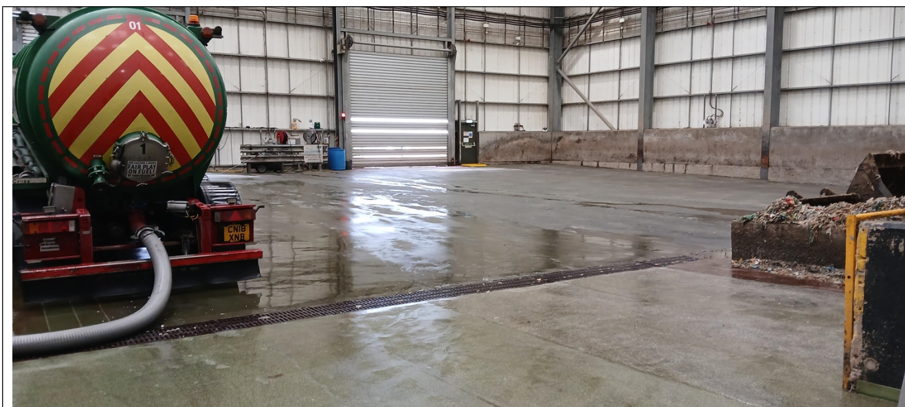
Photo 3 - Waste food reception hall at Severn Trent Parc Stormy
