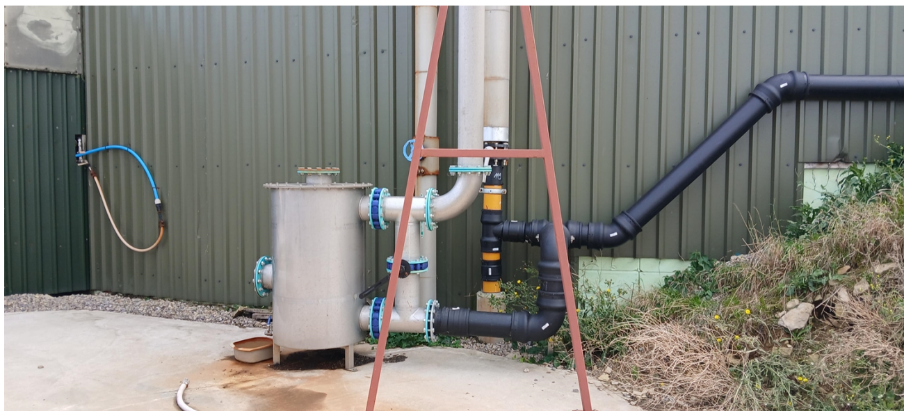
Photo 2 - Newly installed engineering / infrastructure at Pancross Farm
