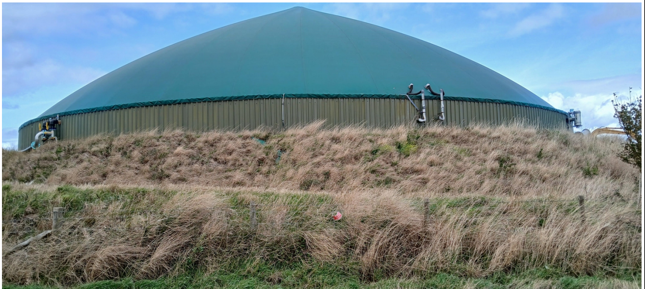
Photo 4 - Digester unit at Pancross Farm with bund
