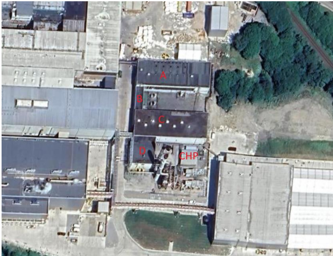
Buildings to be demolished
