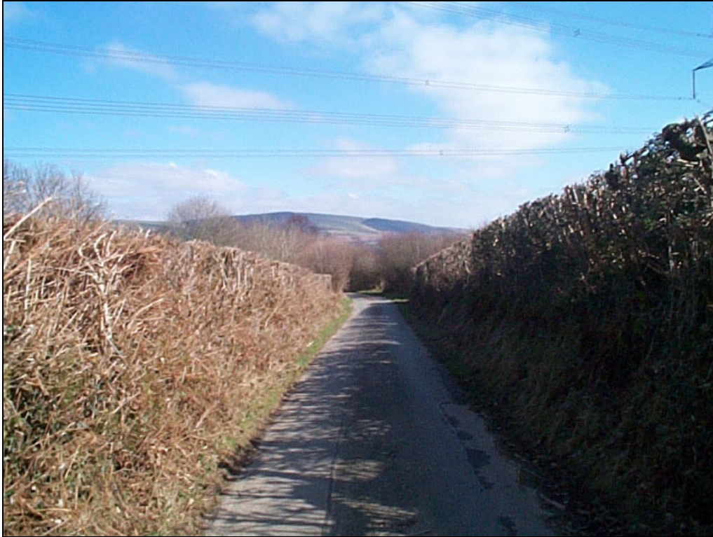
Plate 2: Remains of the DLP embankment
