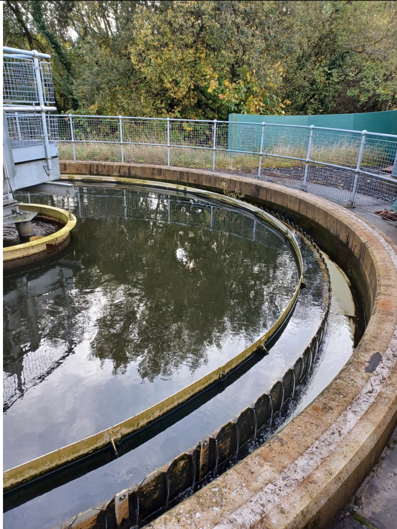
Image 3: Secondary treatment / settlement tank
