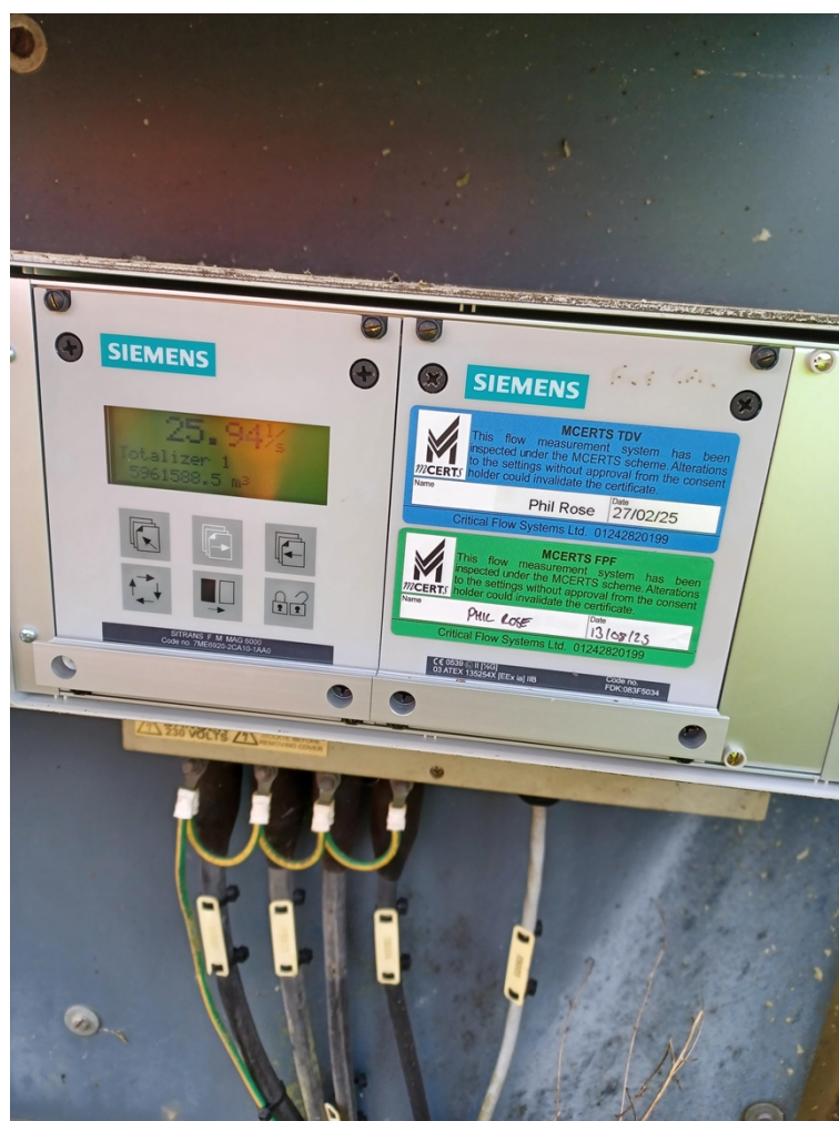
Image 1: flow passed forward meter
