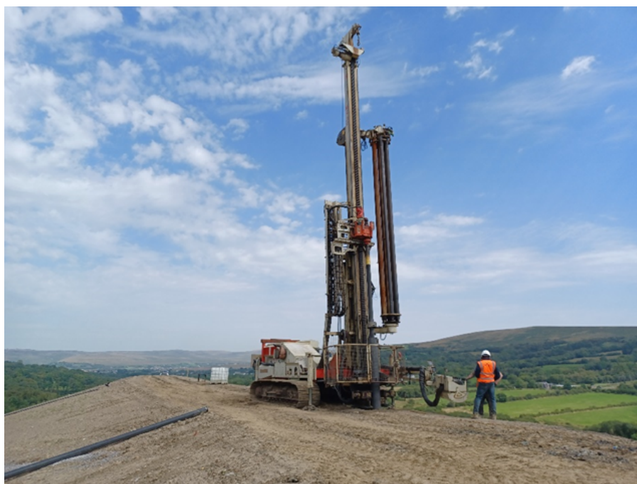
Image 7: Contractors in process of drilling to depth on Peg ID: L3
