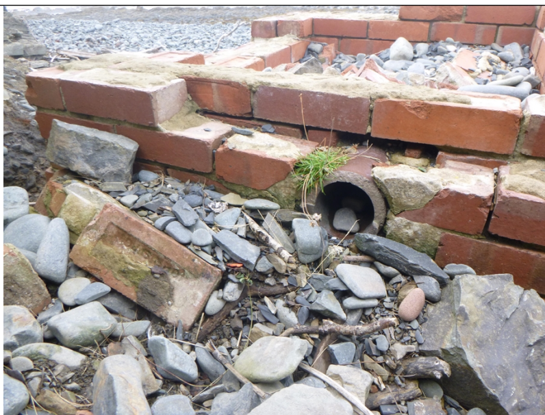
Photograph 6: Pipework leading into disused brick chamber on Tanybwllch Beach at SN 57724 79629
