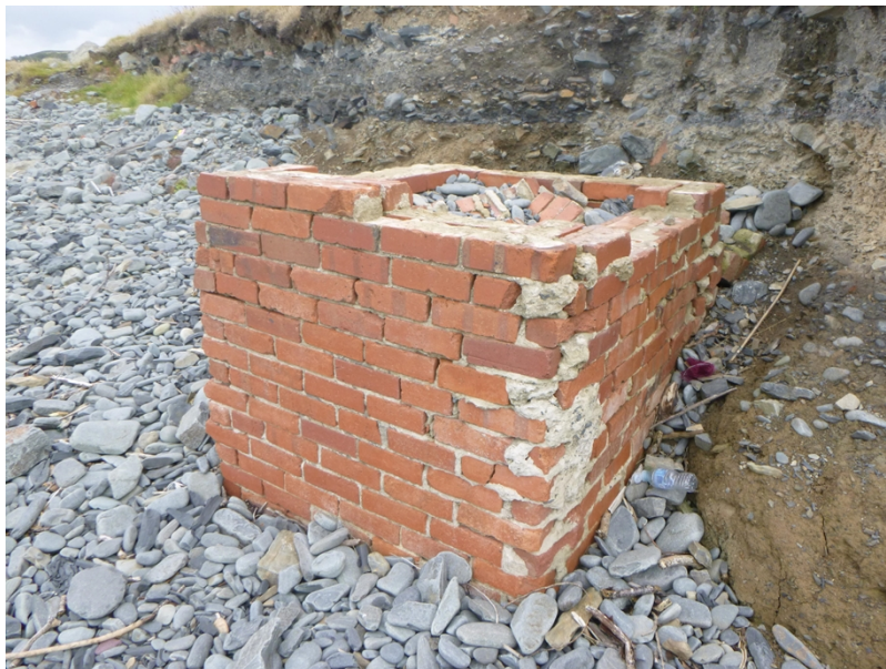
Photograph 5: Disused brick chamber on Tanybwllch Beach at SN 57724 79629
