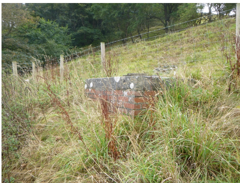
Photograph 7: Brick chamber situated between Plas Tanybwllch's PTP and Tanybwllch Beach at SN 57929 79408
