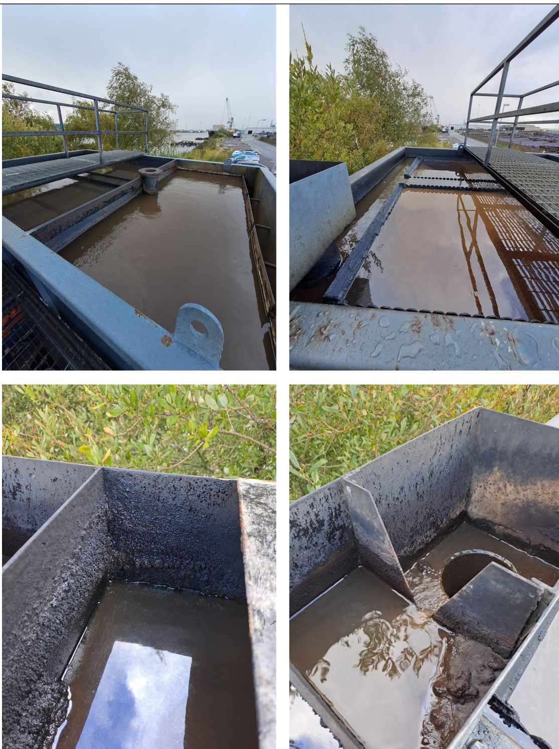
Figure 3 – The treatment system as observed during the visit. Note the presence of minor oil/grease build up on the channel walls.
