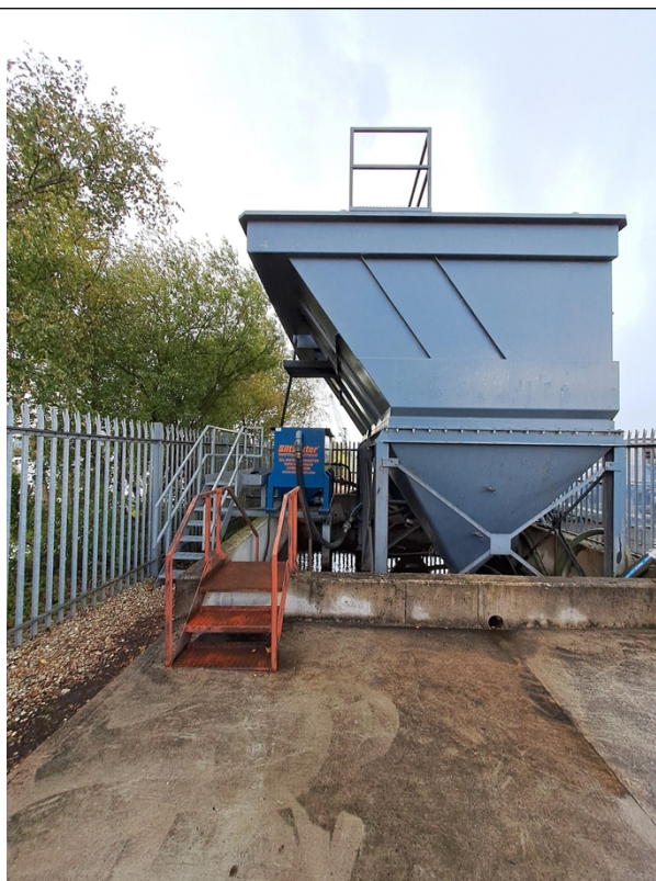
Figure 1 – The general site conditions as observed during the visit.
