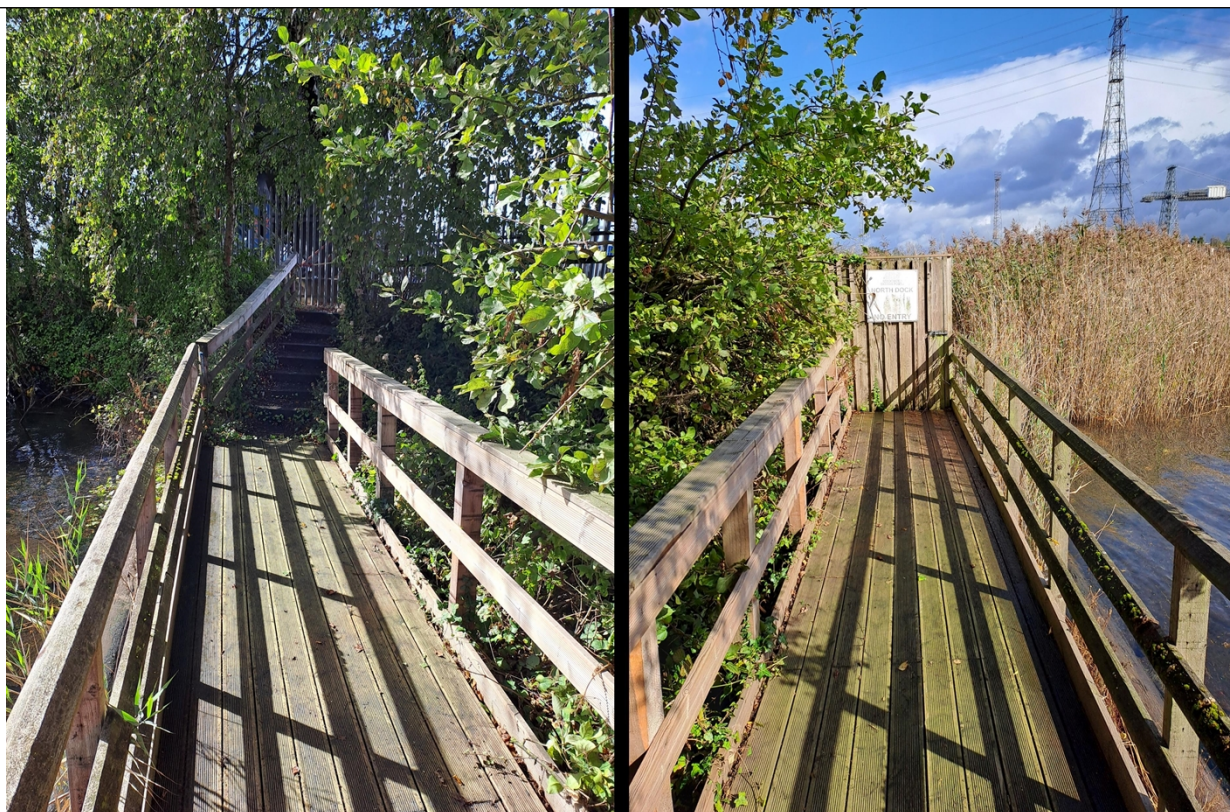
Figure 7 – The access route to the discharge point as observed during the visit.
