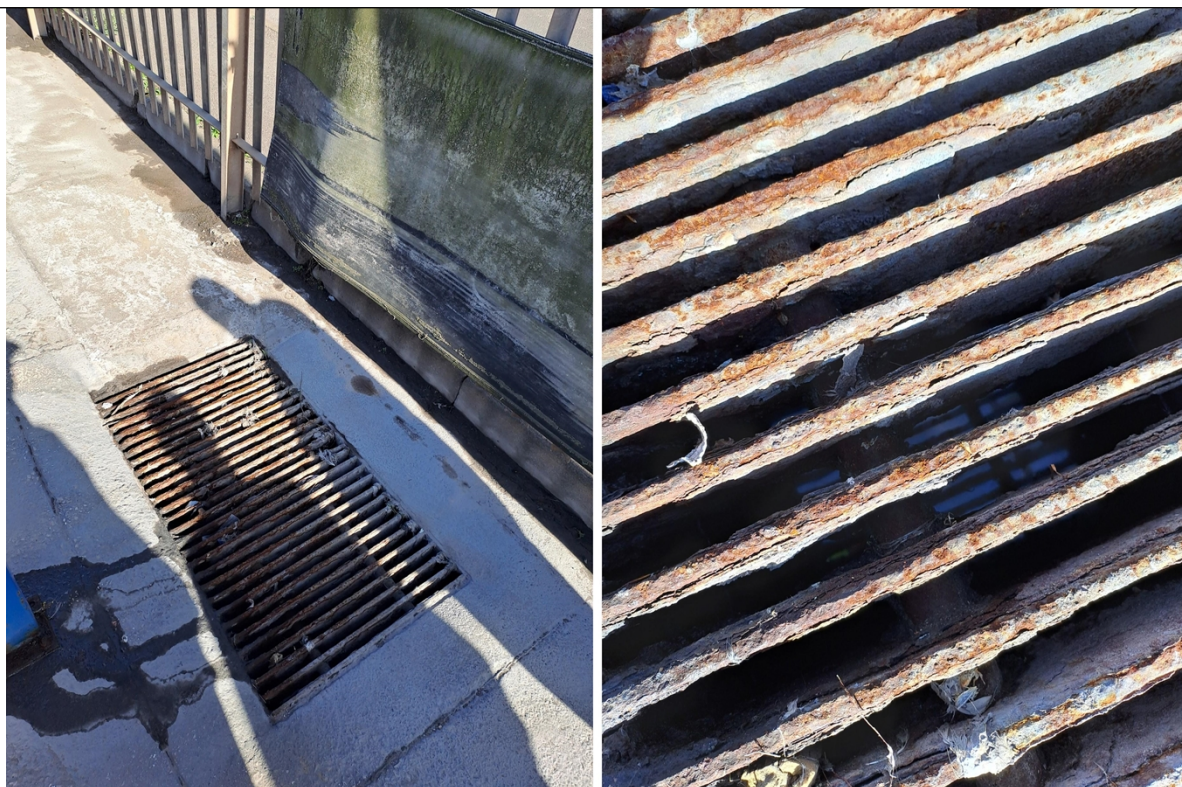
Figure 3 – The sample point/catch pit as observed during the visit.
