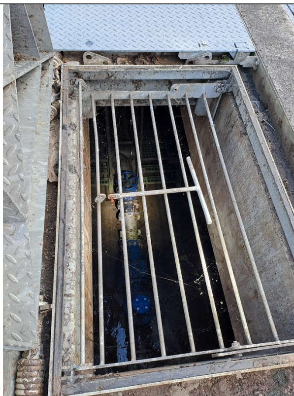
Figure 5: The valve chamber as observed during the visit.
