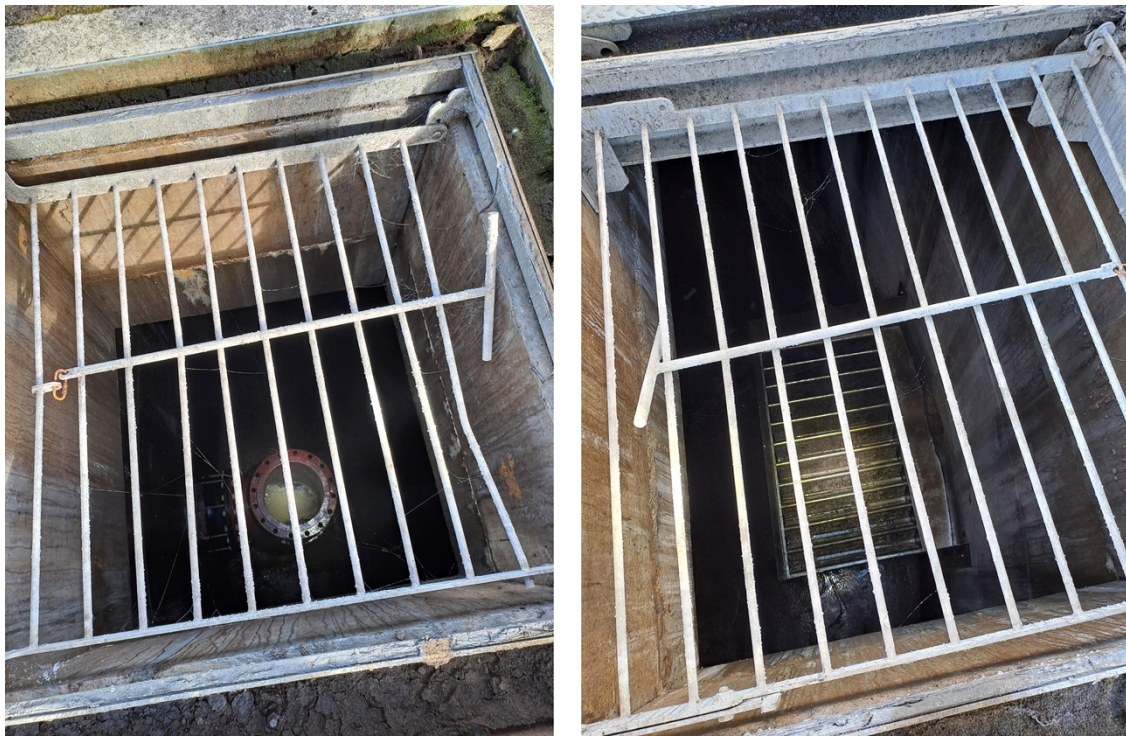
Figure 2: The inlet and screen as observed during the visit.
