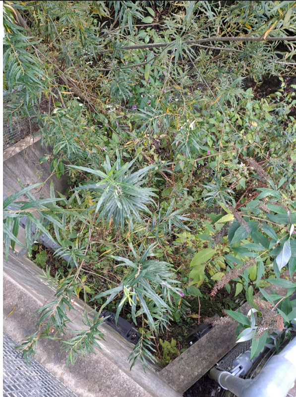
Figure 8: The outfall as observed during the visit.
