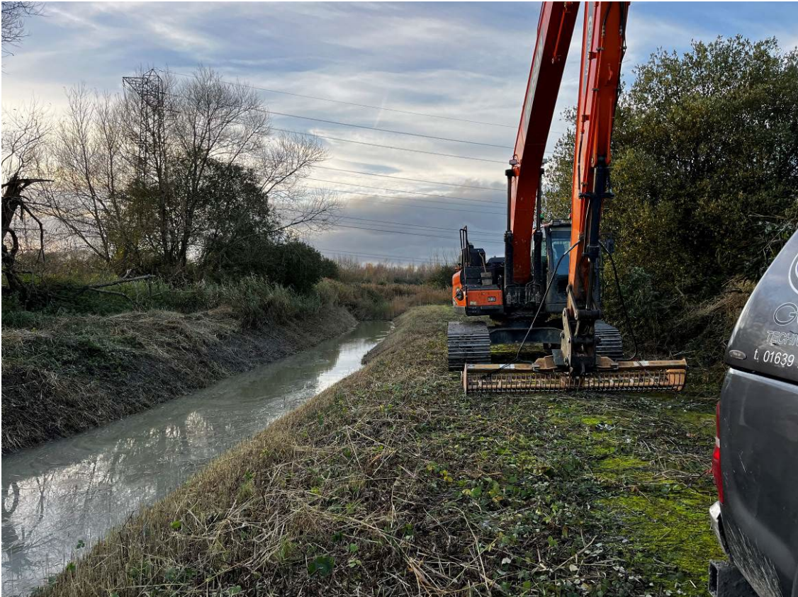
Plate 2-1 Ongoing clearance of inner ditch south of Lagoon 25 (12 November 2024)
