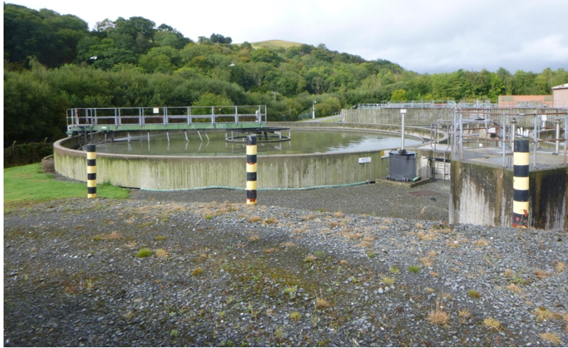
Photograph 3: One of two primary settlement tanks
