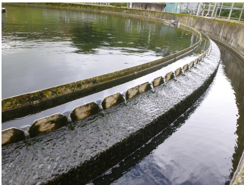
Photograph 6: Discharge from one of three final settlement tanks
