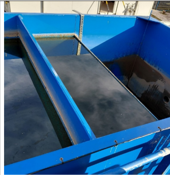
Photo 2. Recently replaced tank.
