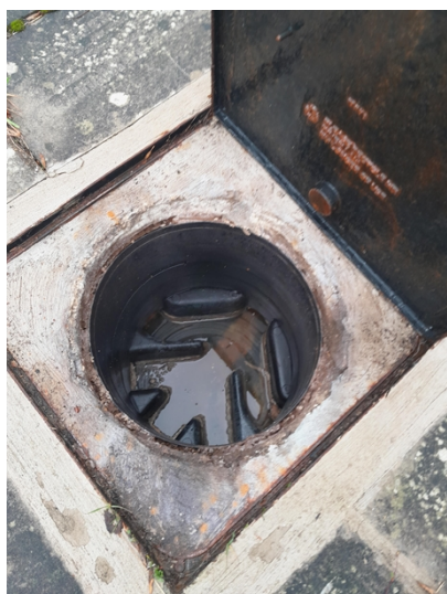
First chamber (Inlet chamber) (Fig 2)
