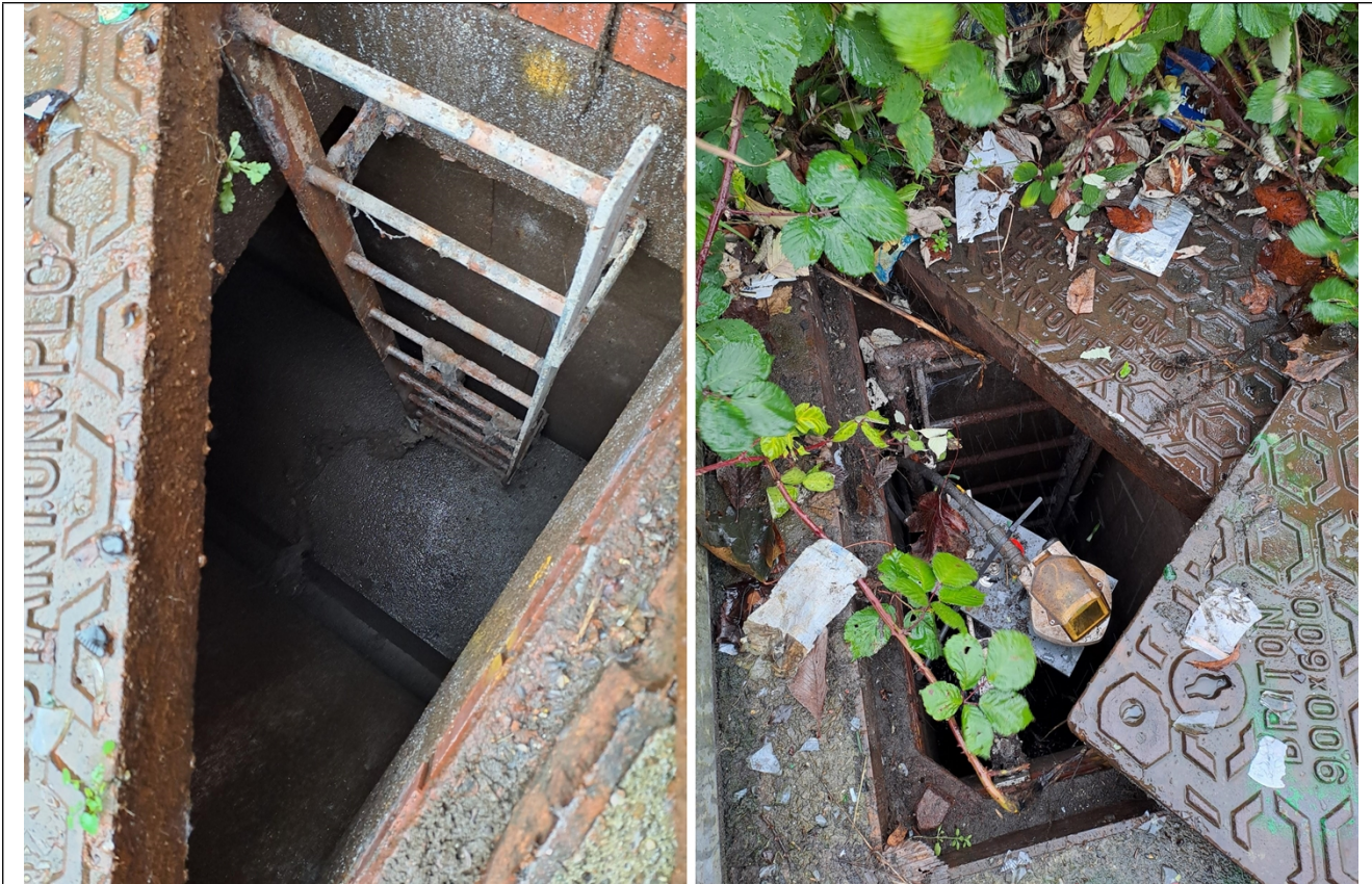
Figure 2: The storm overflow channel and level head sensor as observed during the visit.
