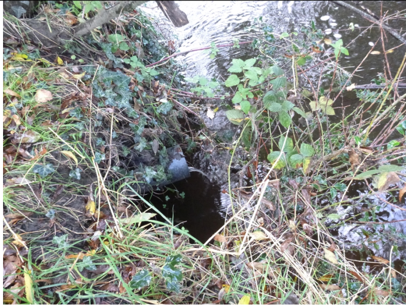
Photograph 2: Outfall into the Afon Aeron
