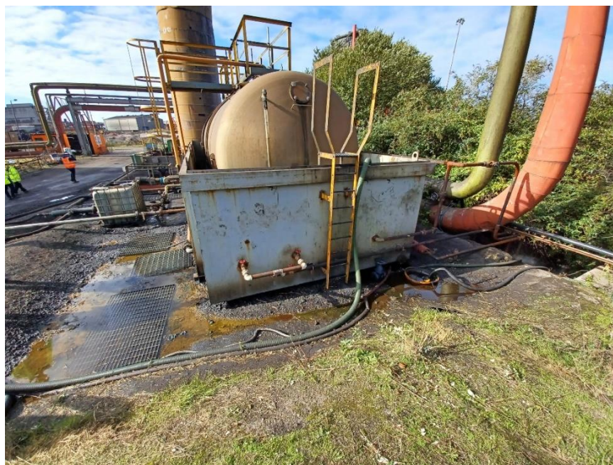
Image 5: Side view of PC1/PC2, oil contaminated surface water within the confines of the "tertiary" containment
