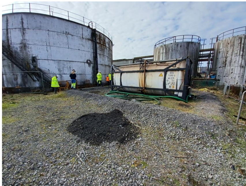
Image 3: Backup oil tank situated within an unlined earth bund, evidence of oil losses outside the curtilage of this earth bunding.
