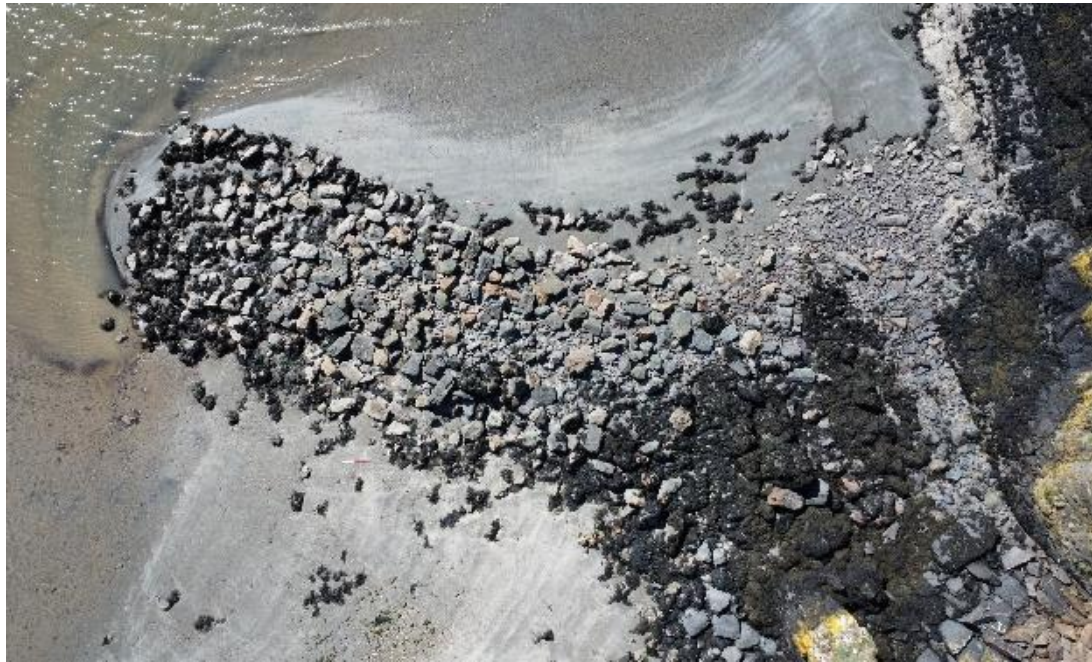
Figure 6. The remains of an historic stone quay at lower town, Fishguard, NPRN 704007 (© Crown Copyright: RCAHMW).
