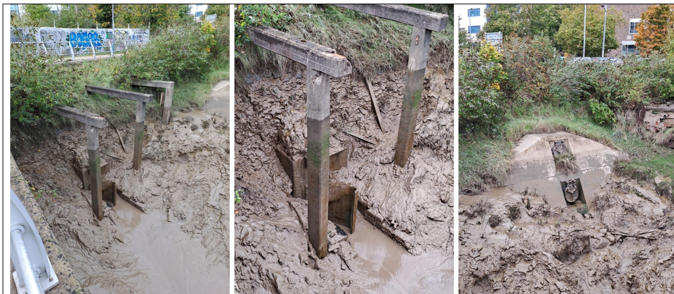
Figure 6 – The outfall as observed during the visit.
