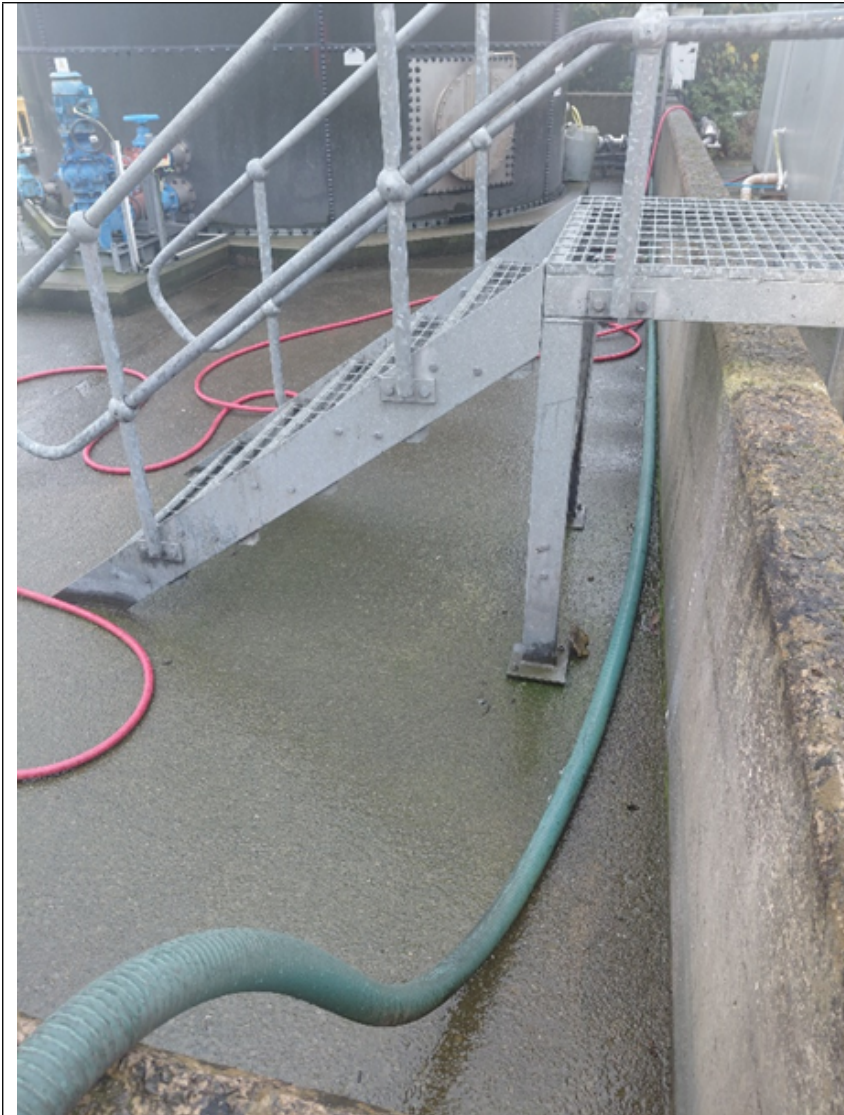
Photo 3. Bunded wall within which the storage tank is located.
