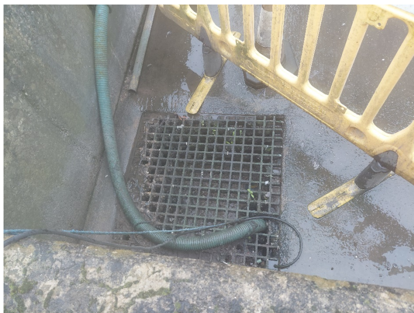
Photo 1. Free flowing drain.
