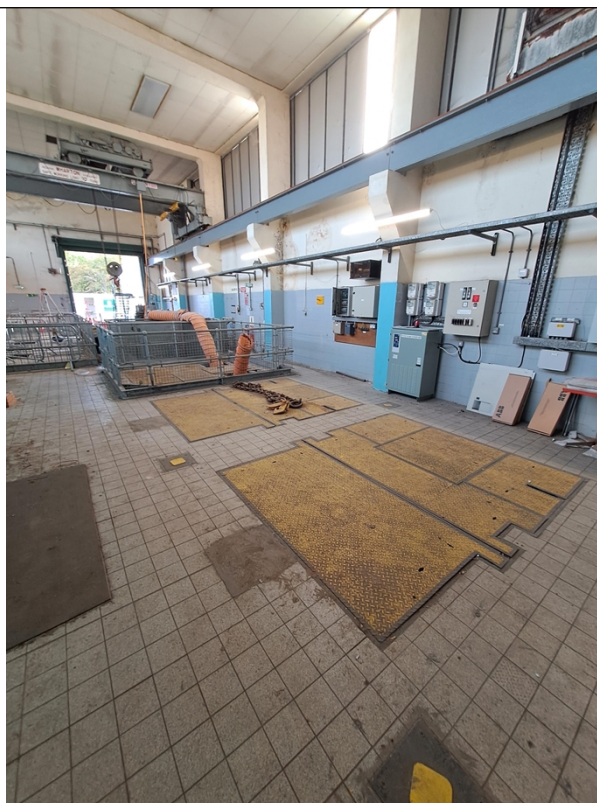
Figure 1 – Control hall conditions at the time of the visit.
