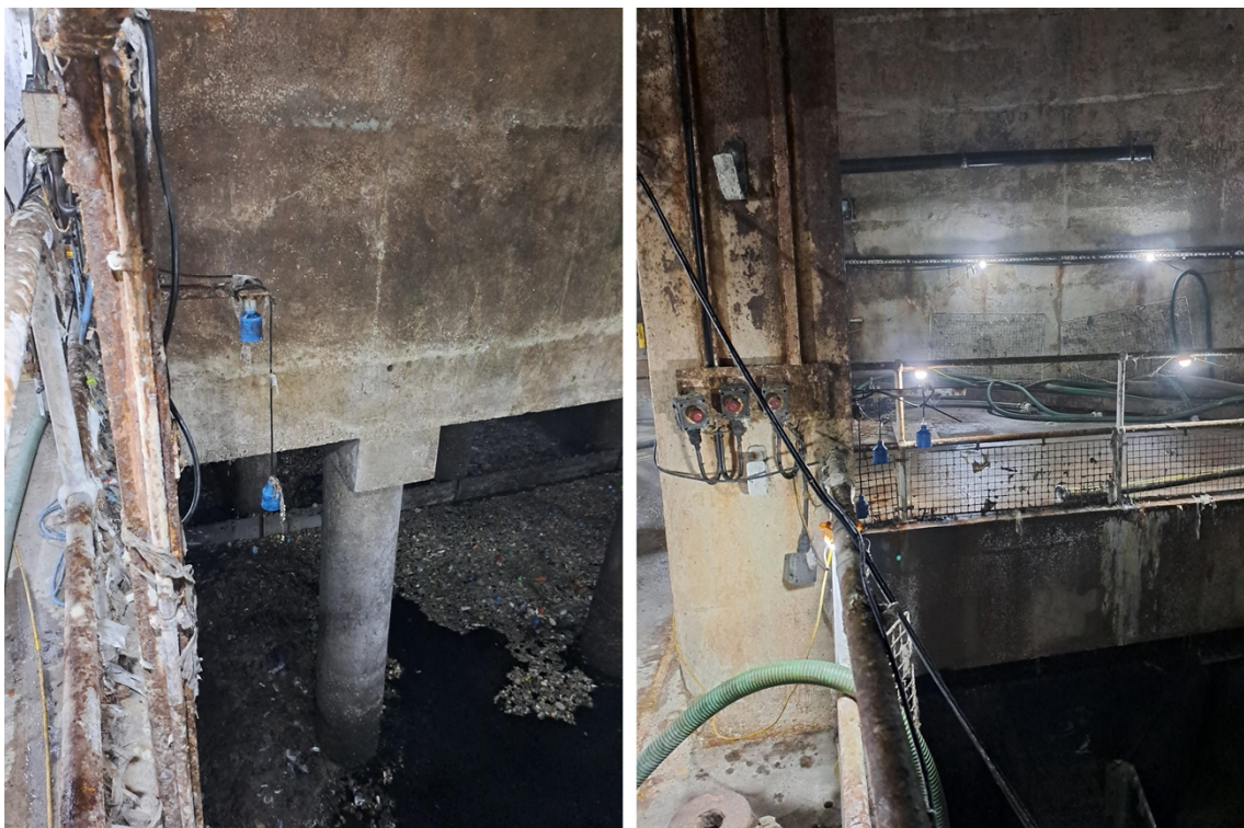
Figure 4 – Level sensor and EDM monitor heads as observed during the visit.
