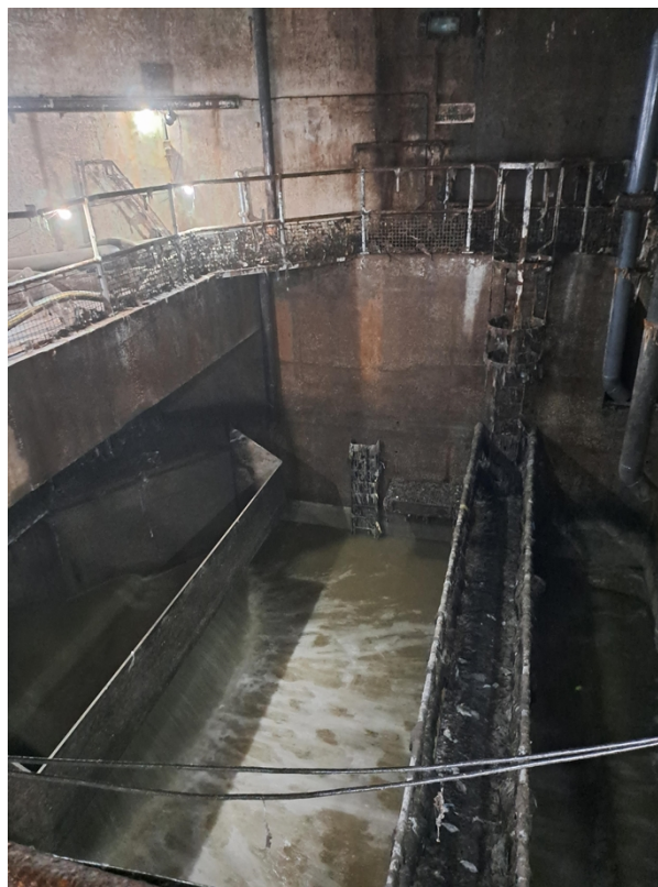
Figure 3 – The wet well as observed during the visit.
