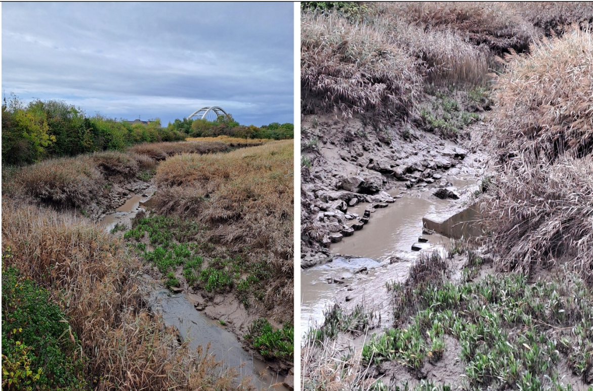
Figure 8 – The outfall as observed during the visit.
