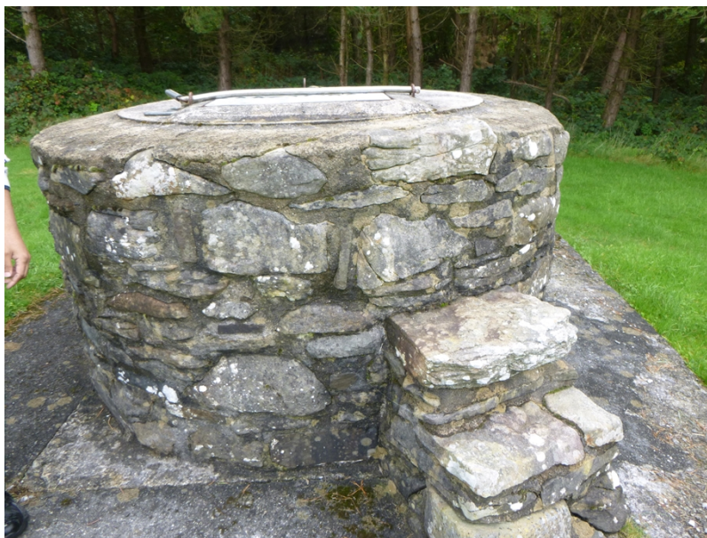
Photograph 1: Borehole at Point A (SN 56278 63052)
