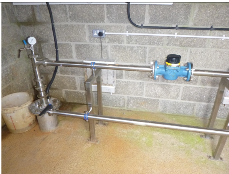
Photograph 3: Borehole and pipework at Point C (SN 55989 63131)
