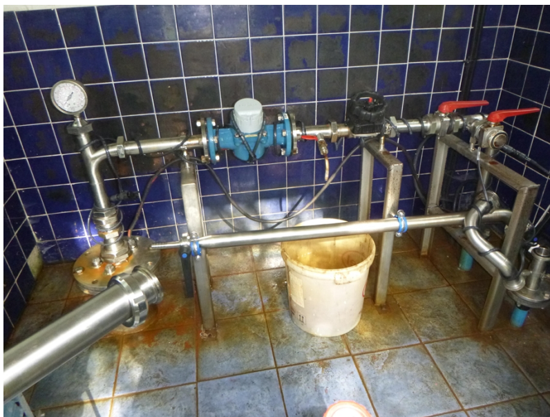
Photograph 2: Borehole and pipework at Point B (SN 56100 63150)
