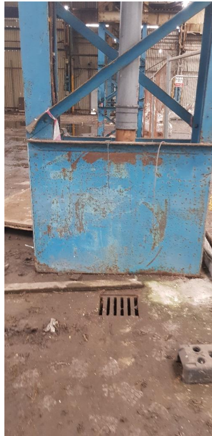
Figure 8 – Existing internal downpipe and floor gully drains.
