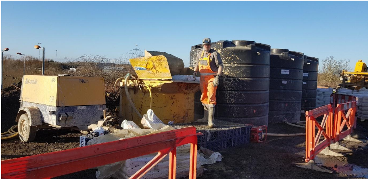
Figure 9 – Typical Treatment Plant setup.
