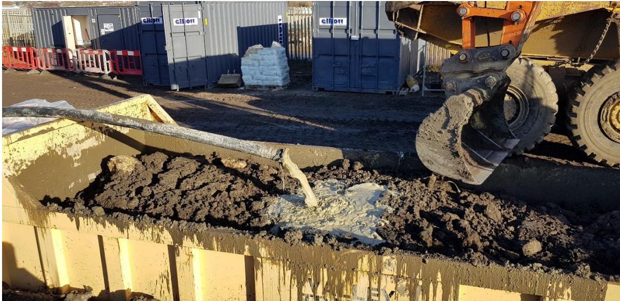
Figure 11 – Soil addition to mixing skip.
