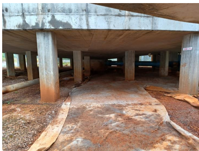
Image 1 & 2 – Liner underneath clarifiers.
