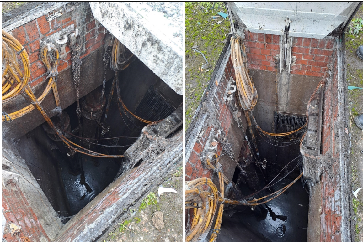
Figure 3 – The wet well as observed during the visit.
