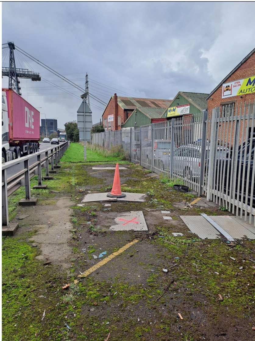
Figure 2 – General site conditions as observed during the visit
