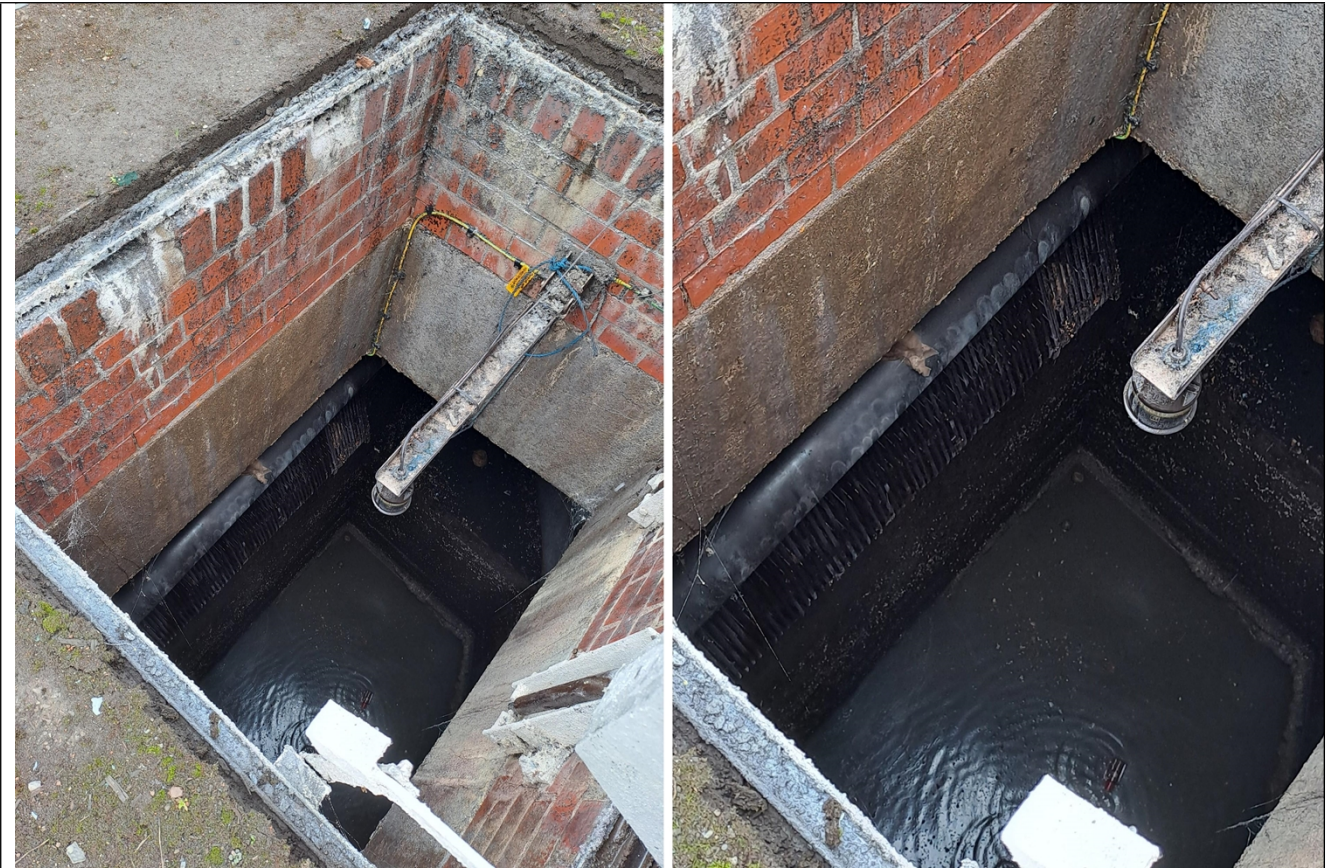
Figure 5 – Apparent presence of a screen within the monitoring chamber prior to discharge, as observed during the visit.
