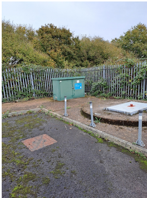
Figure 1 – The general site condition as observed during the visit.
