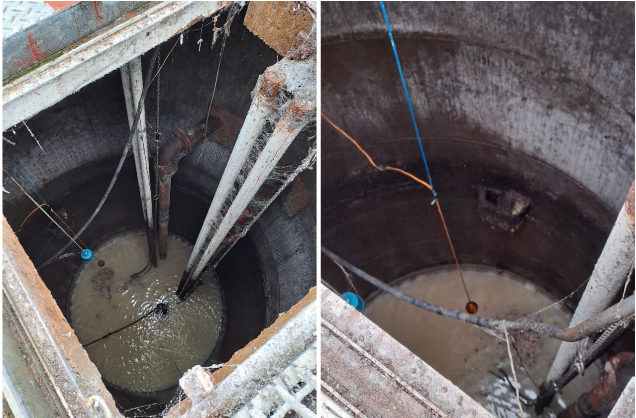
Figure 3 – The wet well conditions as observed during the visit.
