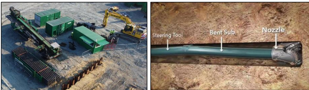
Figure 4.10: Typical drilling rig and pilot drilling assembly
