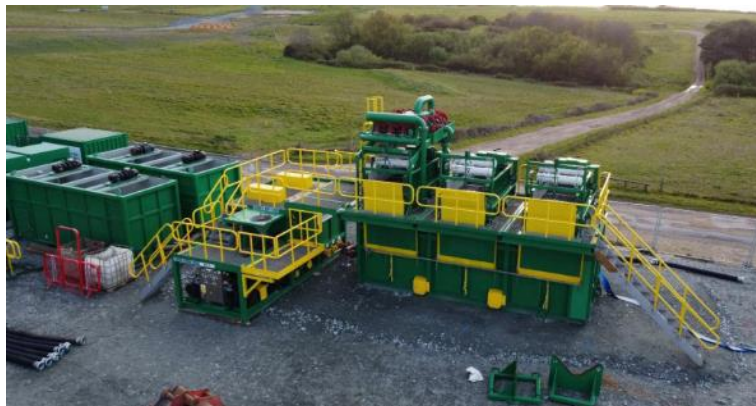
Figure 6.2: Drill Fluid Recycling Plant (typical)
