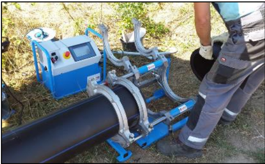
Figure 4.8: Typical pipe welding equipment, storage of pipes and welfare not shown
