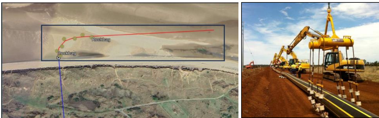
Figure 4.12: Pipe repositioned for pull back
