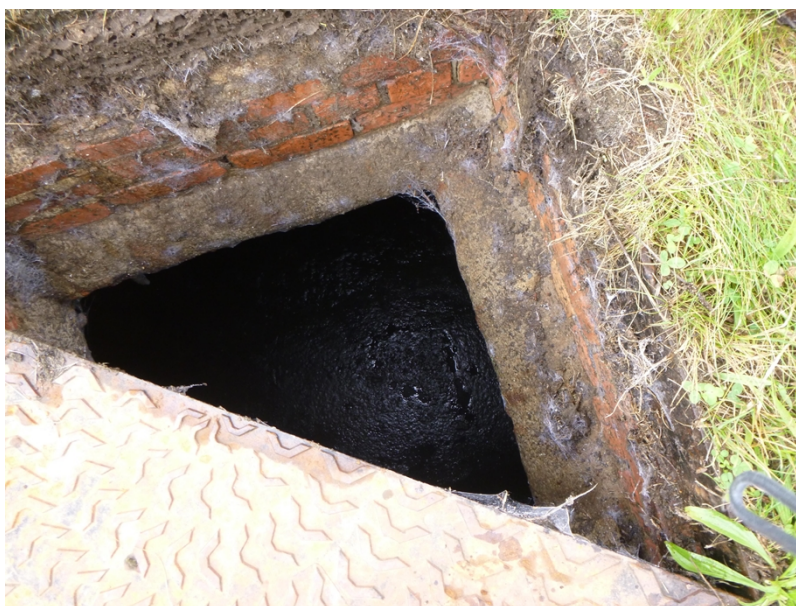
Photograph 3: Entry into storm tank
