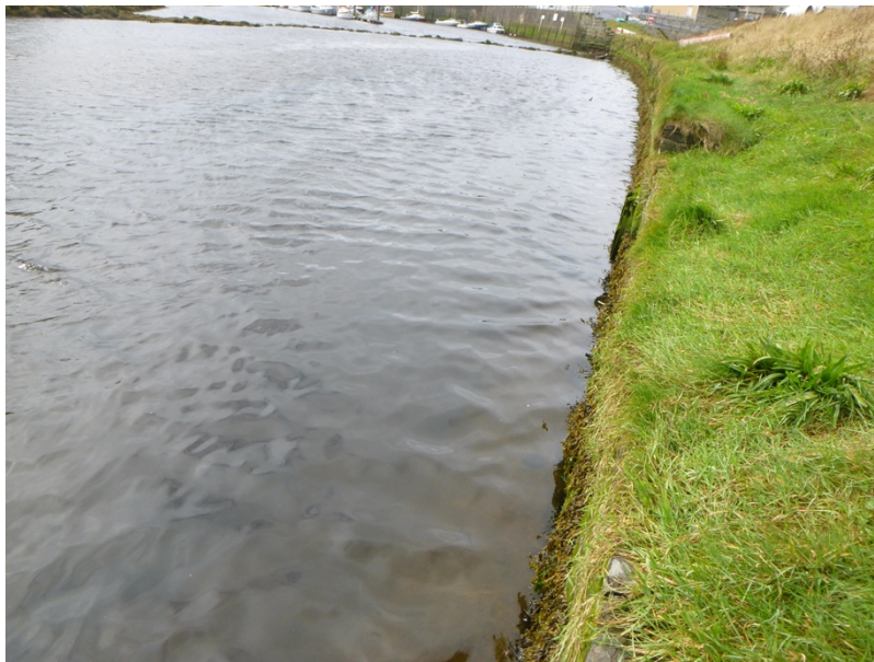
Photograph 6: Suspected emergency outfall into the Afon Rheidol
