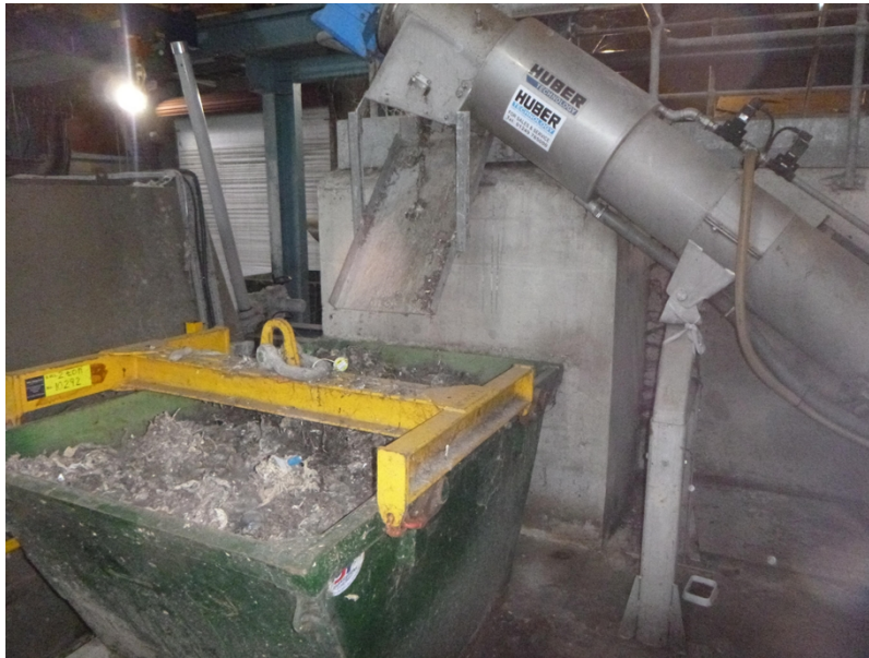
Photograph 2: Screenings deposited into skip
