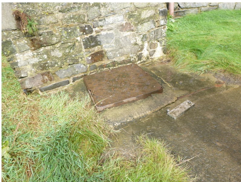
Photograph 5: Storm and settled storm sample point
