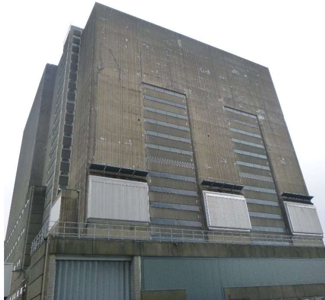
Figure 2: Reactor Building 2 - South Elevation
