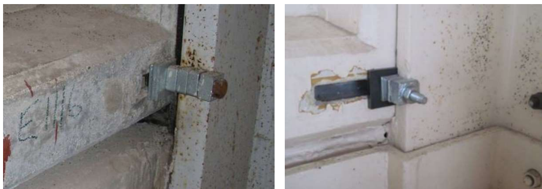
Figure 15: Example Lindaptor Repair
