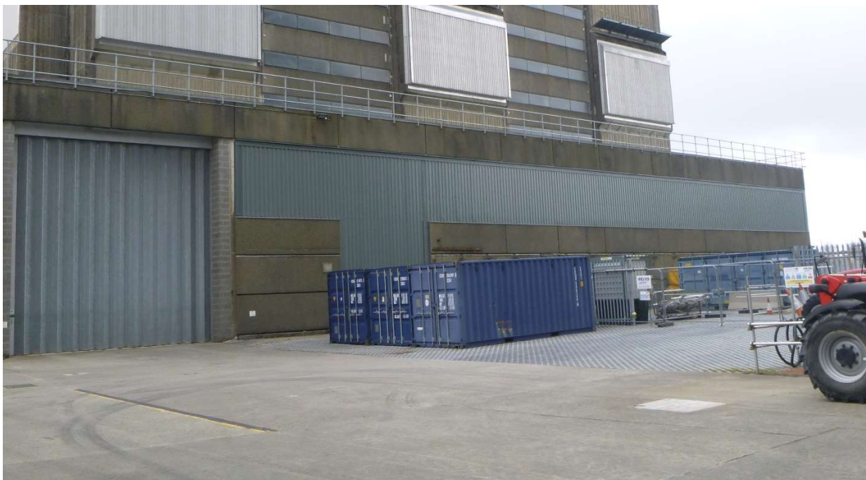
Figure 1: Reactor Building 2 - South Gas Circulator Hall
