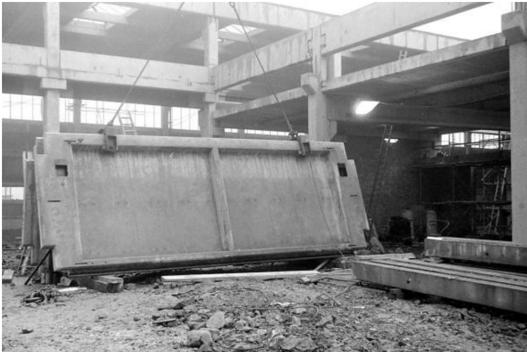
Figure 10: Typical PCCP lift set up
