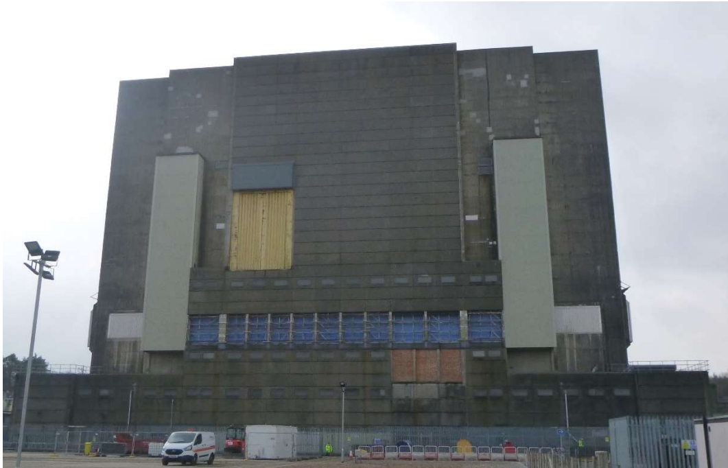
Figure 4: Reactor Building 1 - East Elevation
