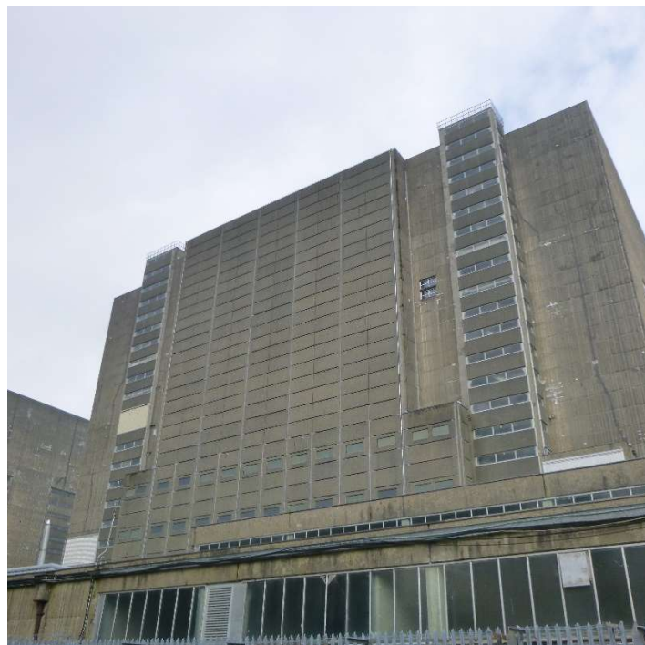
Figure 3: Reactor Building 1 - West Elevation
