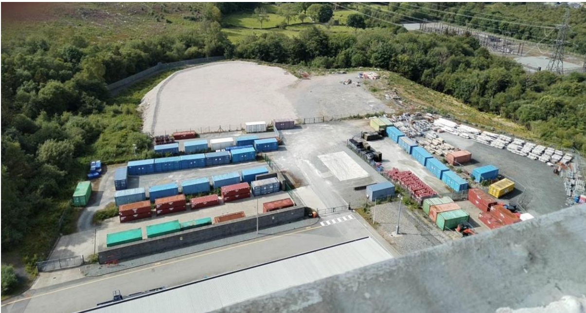
Figure 10 – RCA laydown area (2024)
