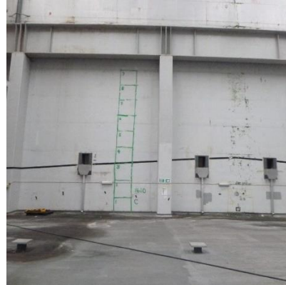
Charge Hall with 1 x 9 metre strip for surveying
