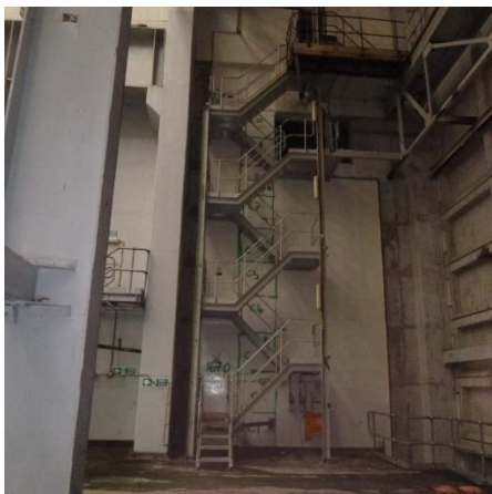
FMMB with 1 x 10 metre strip for surveying
