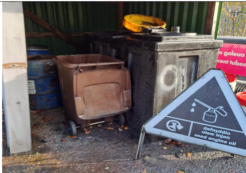
Image 5 Shows the containment area for waste oil in line with permit conditions.
