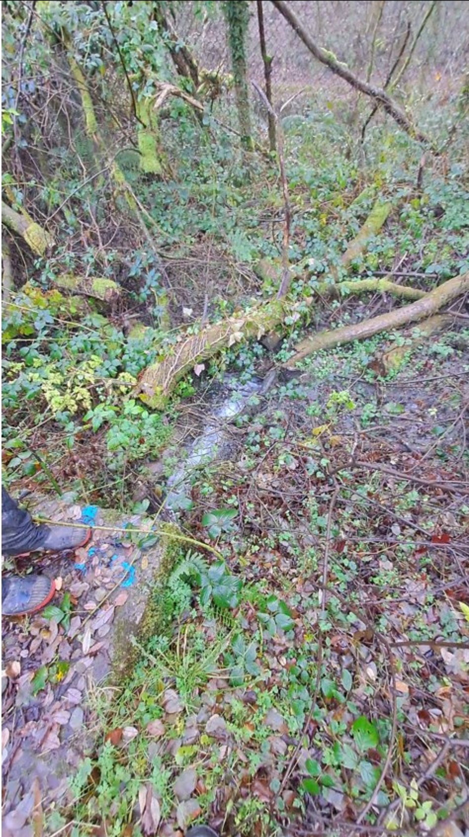
Figure 2 Channel before final effluent discharge point was overgrown
