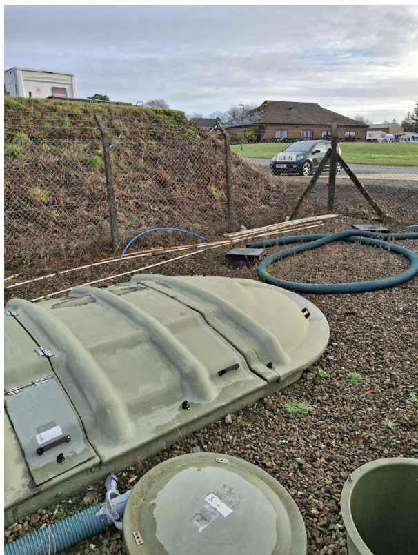
Fig1: External view of system one
