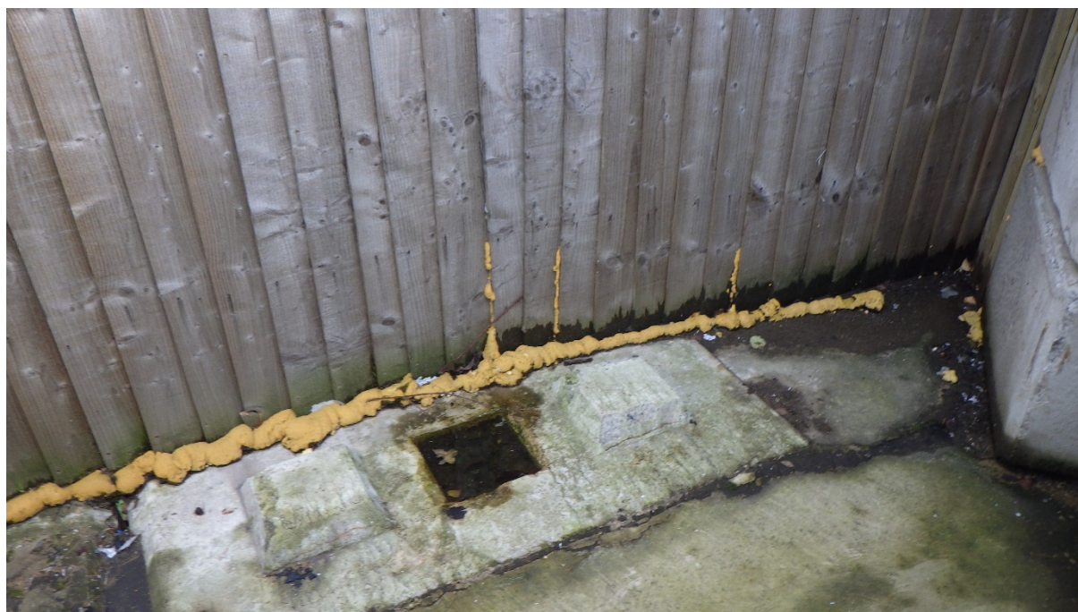
Acoustic wall sealed.
