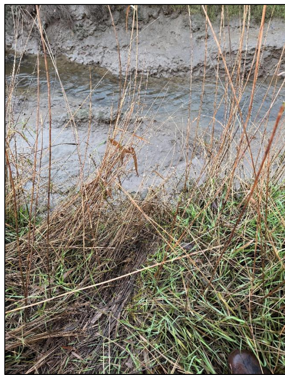
Figure 5: Potential mammal path on the East side of the culvert.
