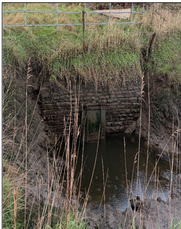
Figure 4: Vegetation around the East side of the culvert.
