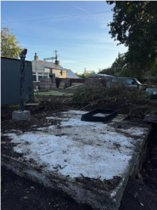
Pic 2 Cesspit Tank
