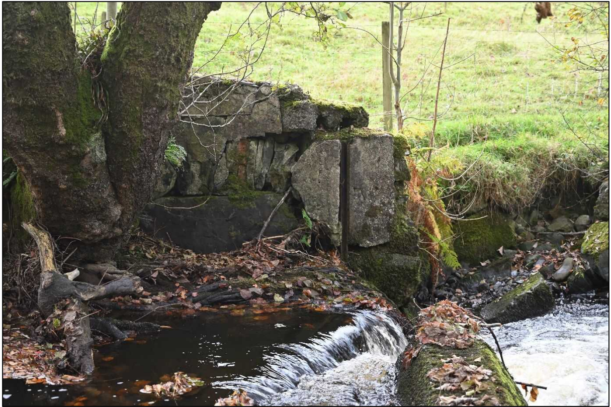
Plate 5: Sluice, looking south
