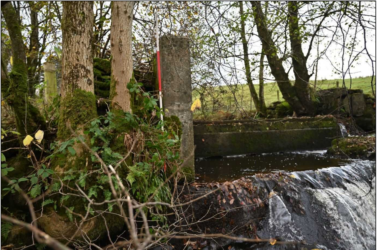
Plate 14: End of the concrete head wall on the northern side of the river
