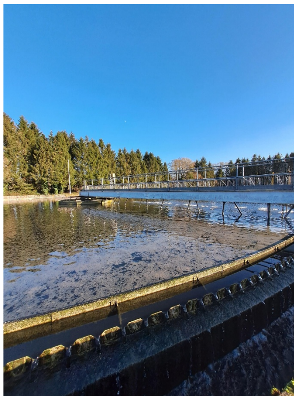
Figure 19 – An example of the pin floc observed in the final settlement tanks during the visit.
