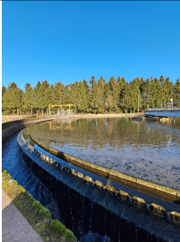
Figure 21 (Bottom) - Final Settlement Tank 2 as observed during the visit.
