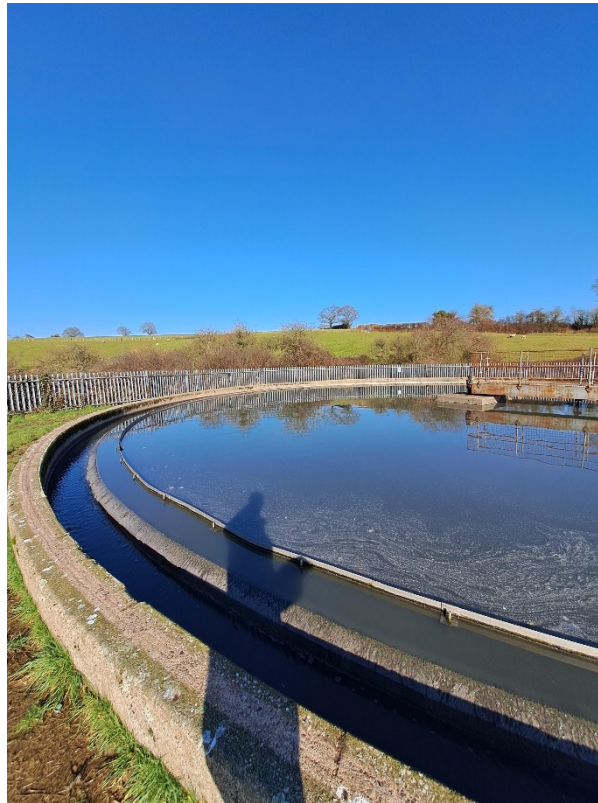
Figure 15 (Top) – Condition of Tank 6 as observed during the visit.
