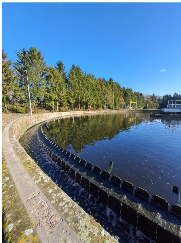
Figure 20 (Top) – Final Settlement Tank 1 as observed during the visit.
