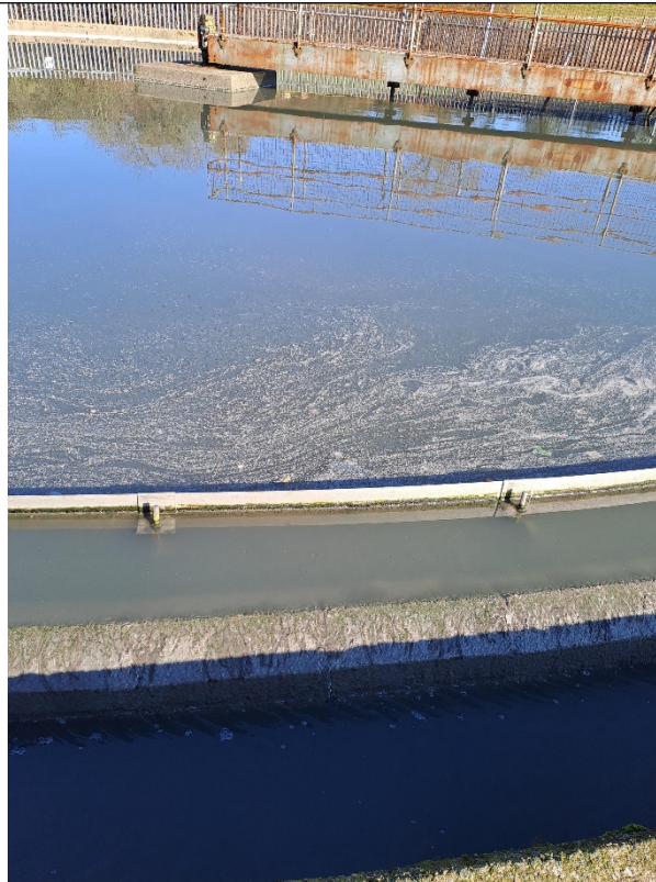
Figure 16 (Bottom) – Tank 6 baffles in very good condition.
