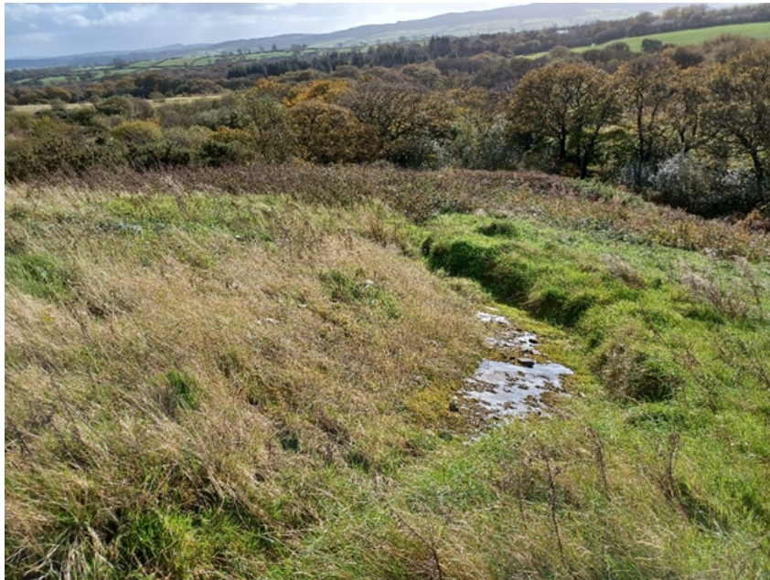
Image 5: Evidence of slope failure noted on SW flank of Cell 4.
