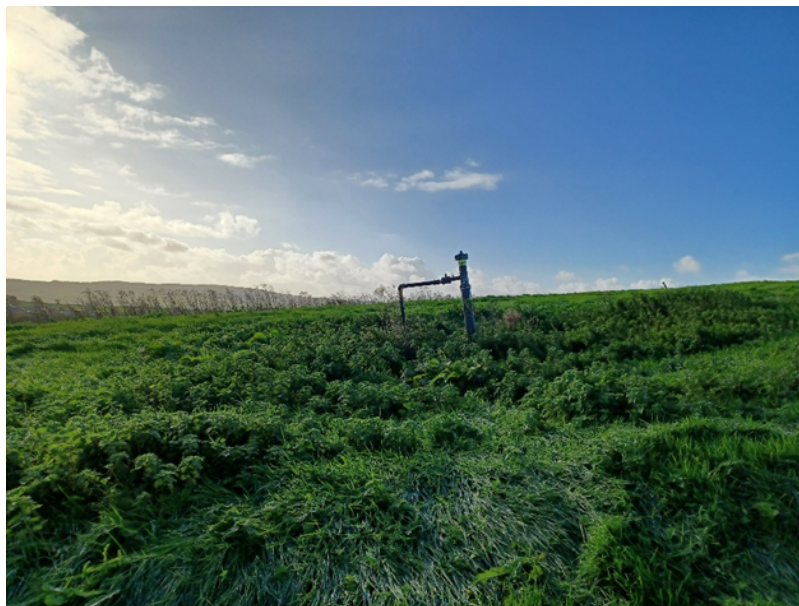
Image 1: Example of subsidence around NYCW1103.
