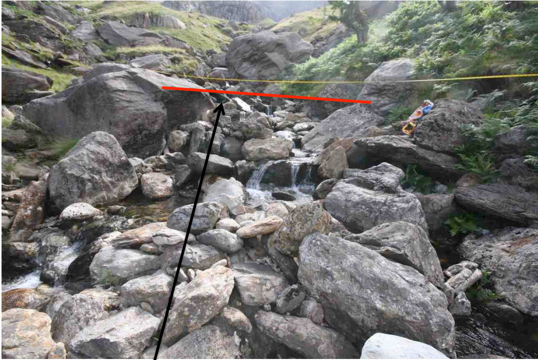
Weir crest line, shown in red, below series of natural steps
