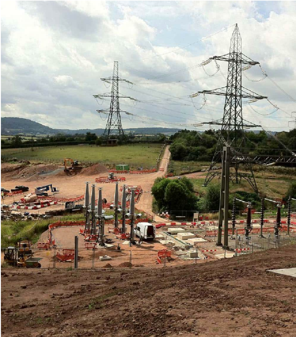
The undergrounding of electricity cables at Ross-on-Wye
